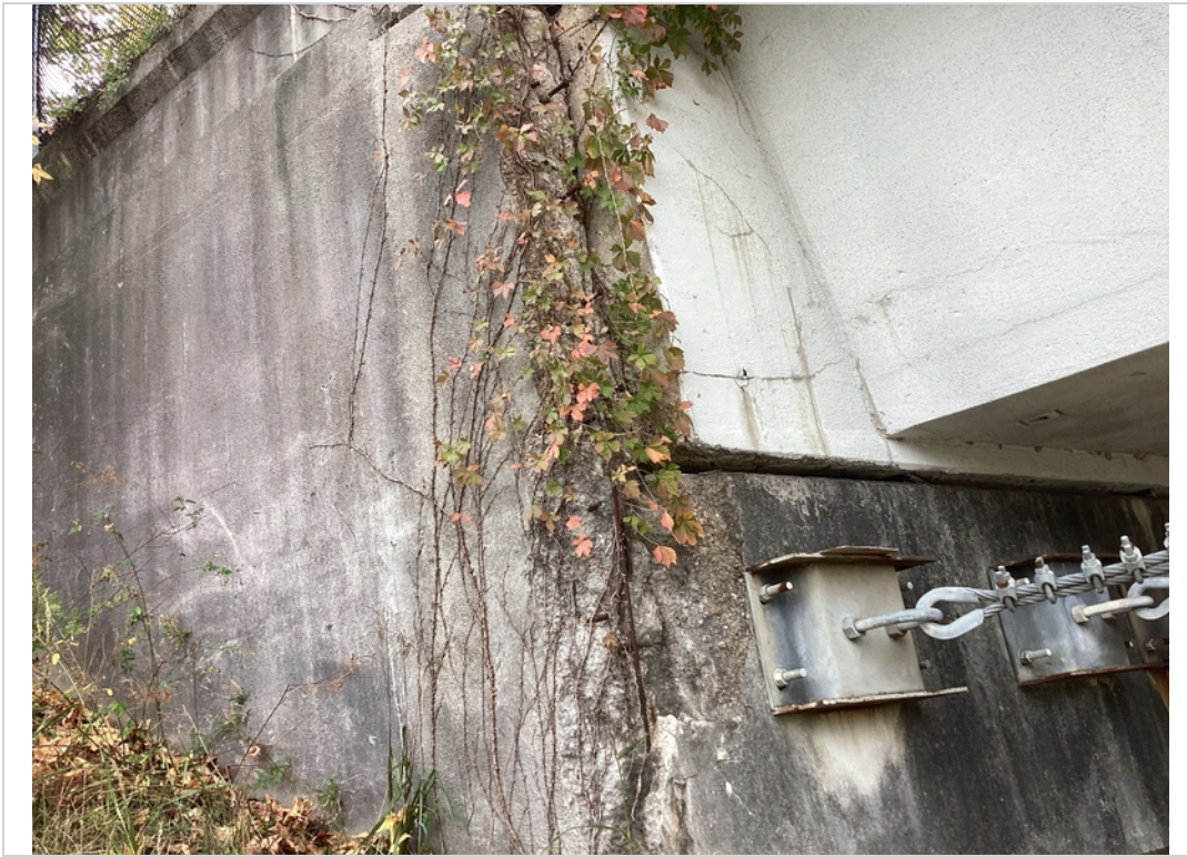
Abutment 2/left wing spall to steel
