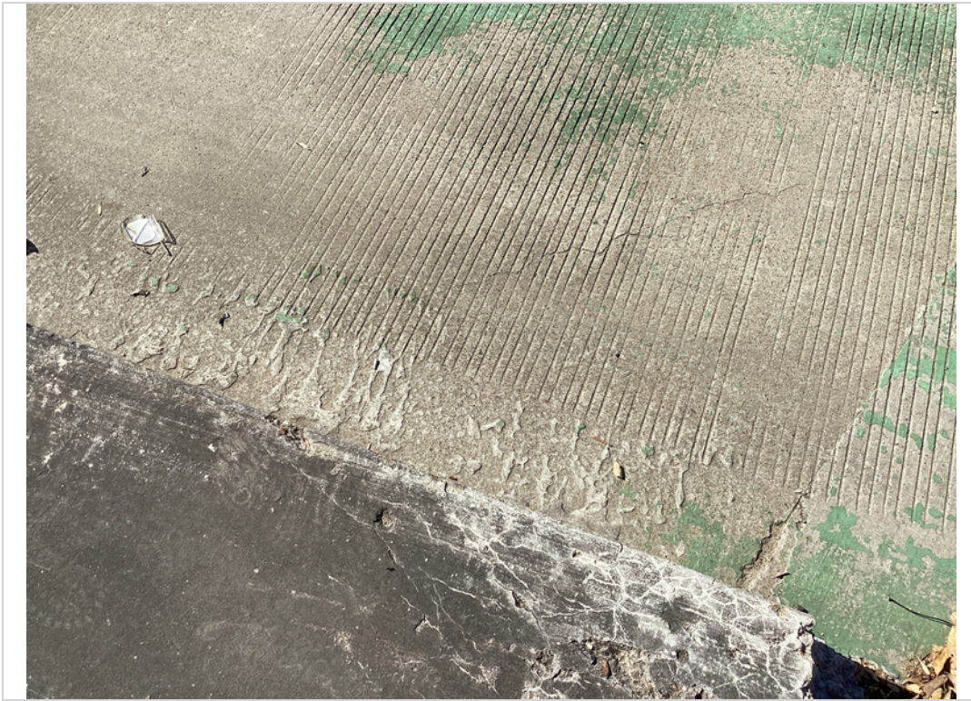
Span 1 , cracks & sidewalk light scaling
