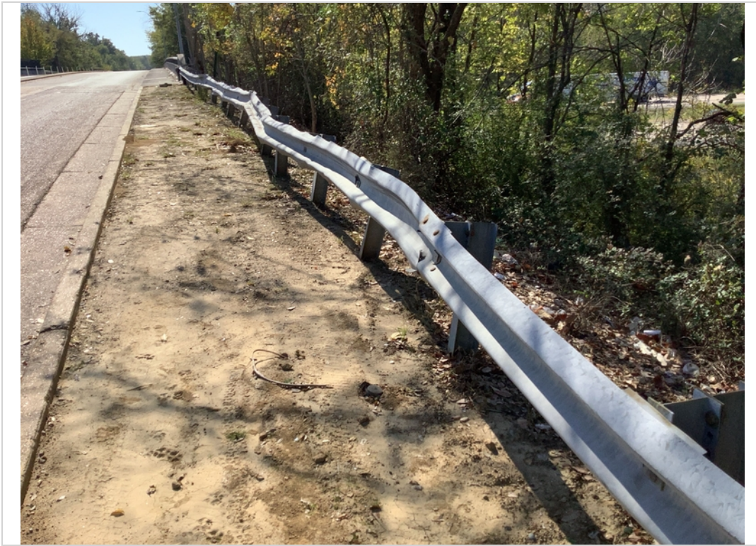
Approach 1 right guard rail collision damage
