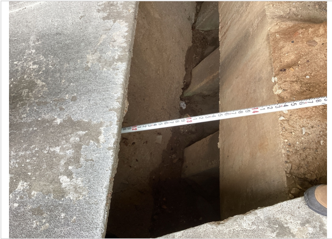
Washing below slope paving at abutment 2
