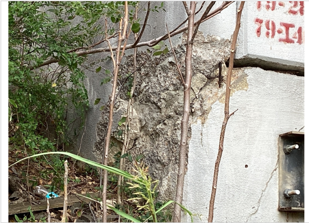
Abutment 1 spall to steel
