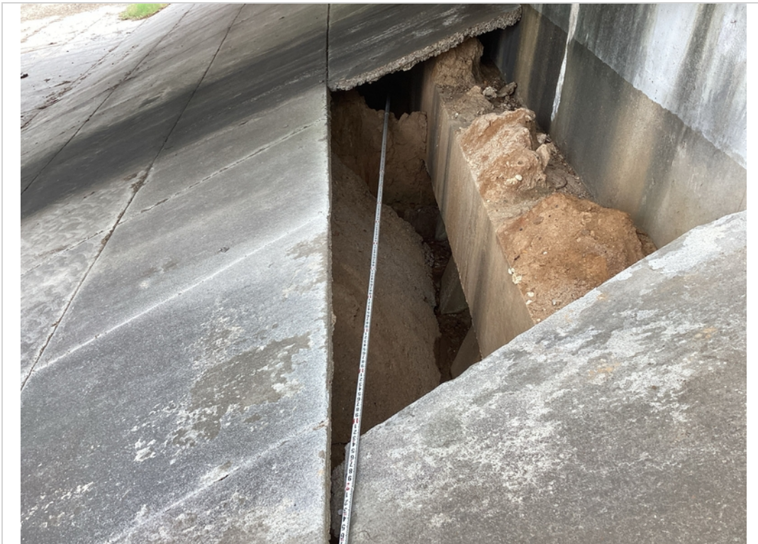
Washing below slope paving at abutment 2
