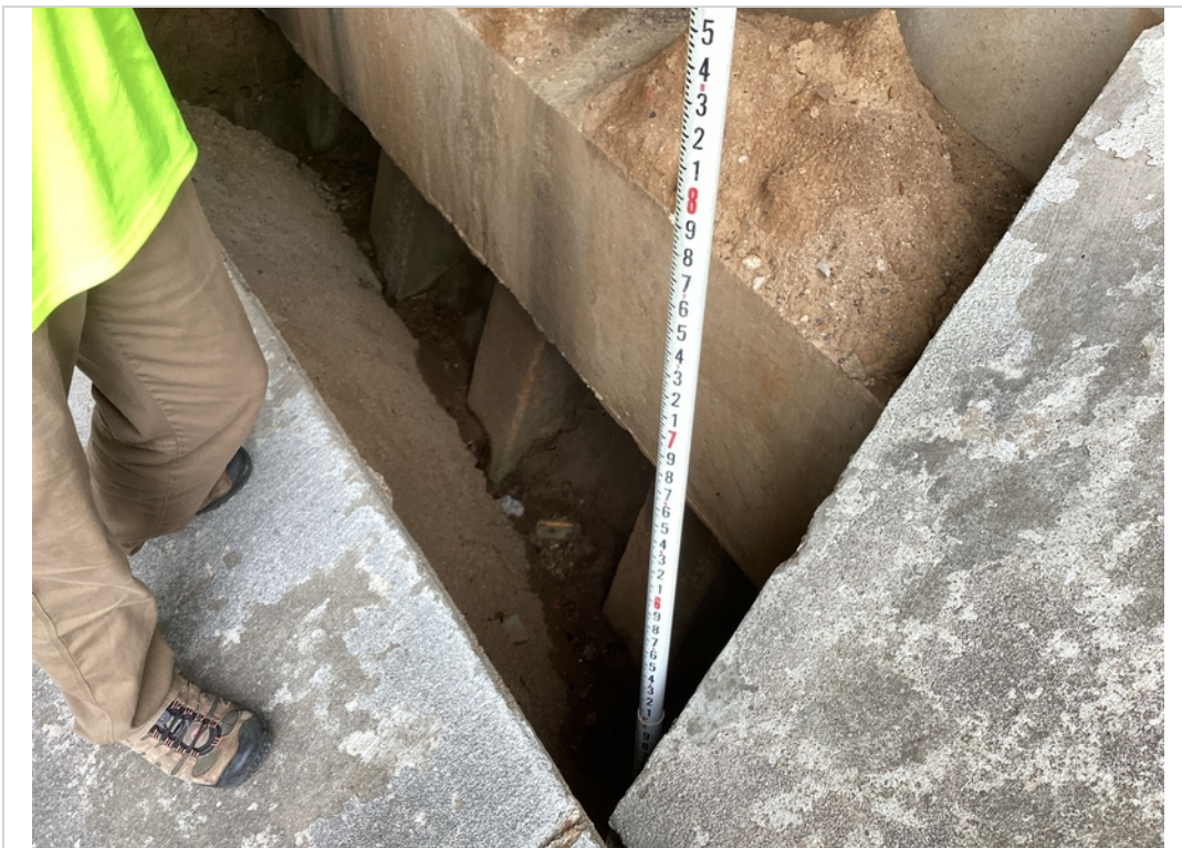
Washing below slope paving at abutment 2
