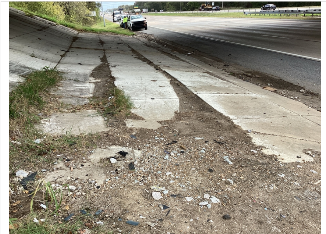
Abutment 1 slope paving sinking/bucking
