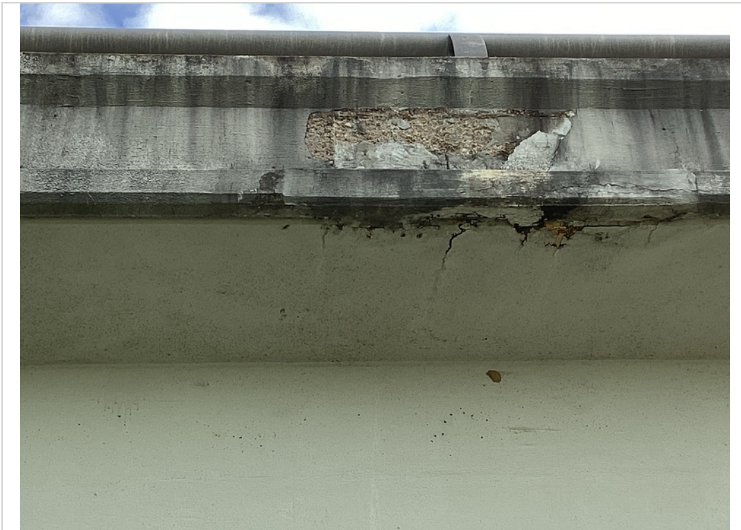
Span 1 overhang spall
