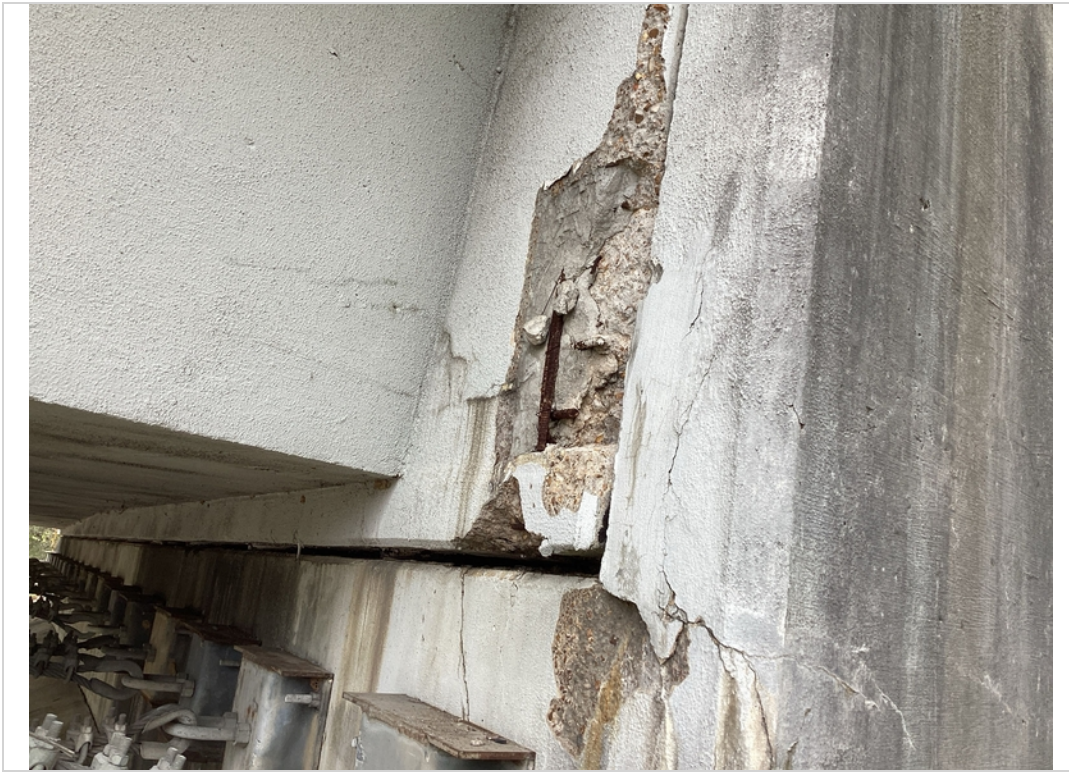
Abutment 2 backwall spall to steel
